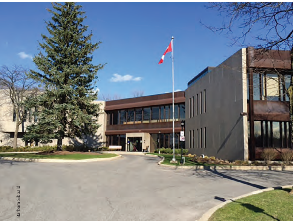
CMA House, a 43 000 square foot modernist structure which opened in 1970, was demolished in 2016 due to high renovation costs. A new structure was slotted to be built.
